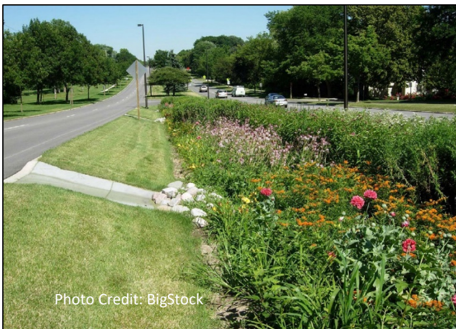
A vegetated Bioswale which reduces storm water runoff, erosion and provides pollinators with habitat.
