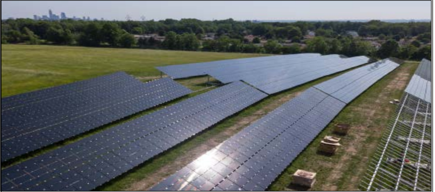
Solar Panel Installation on Brooklyn Brownfields, Cuyahoga County. This 4.0 MW array was constructed on approximately 17 acres of a 75-acre former landfill site and is designed to generate over 5,000,000 kWh of electricity annually. It can provide approximately 8% of the electrical consumption for 10 County-owned buildings (Resource from the CCCCAP).
