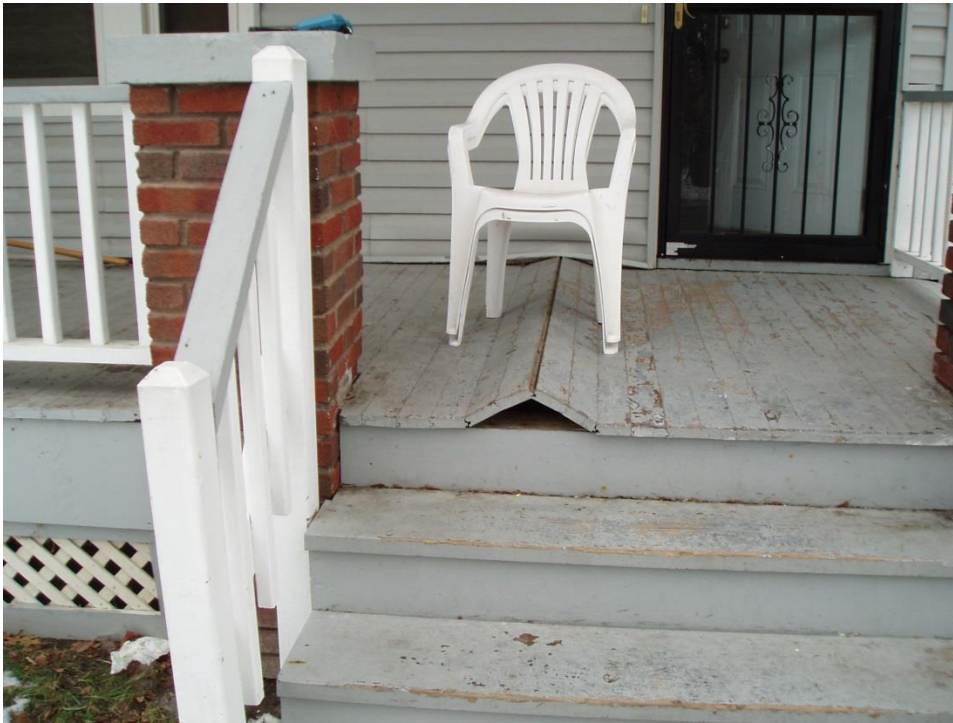
Warped Floor
