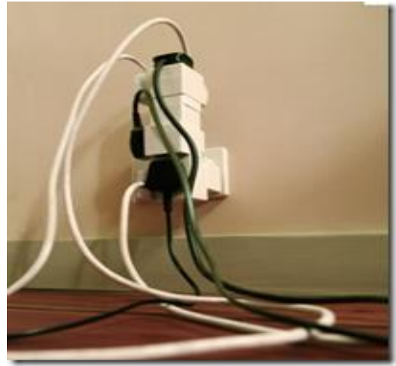
Overloaded Circuit
